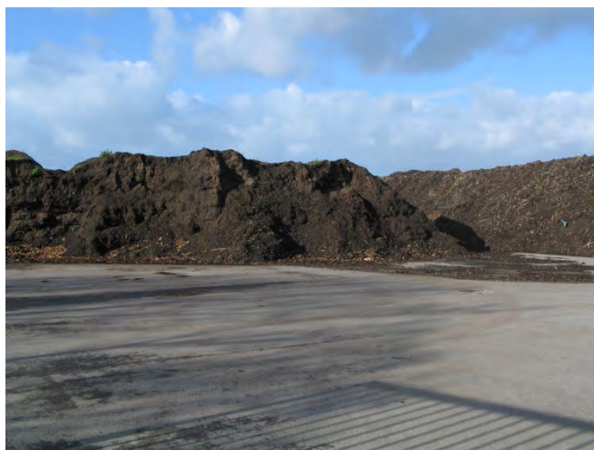
Station de co-compostage (Plonévez-Porzay/Croix-Neuve)
